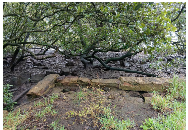
Sandstone block remnants of the old Henley Pleasure Ground boatshed (image above)
